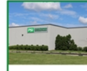
PSI R+D, Engineering & HD Assembly Facility 1465 Hamilton Pkwy. Itasca, IL 198,000 sq. ft.
