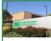
PSI Corp. HQ & Engine Dress Facility 201 Mittel Dr. Wood Dale, IL 261,000 sq. ft.
