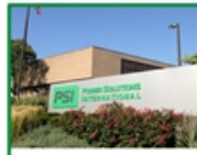
PSI Corp. HQ & Engine Dress Facility 201 Mittel Dr. Wood Dale, IL 261,000 sq. ft.
